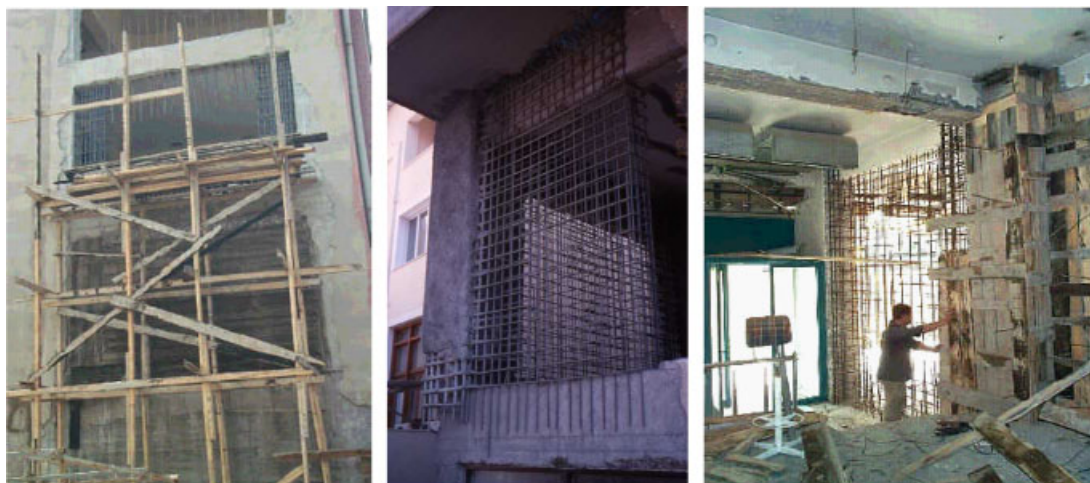
Fig. 5 Cast-in-place infill walls
