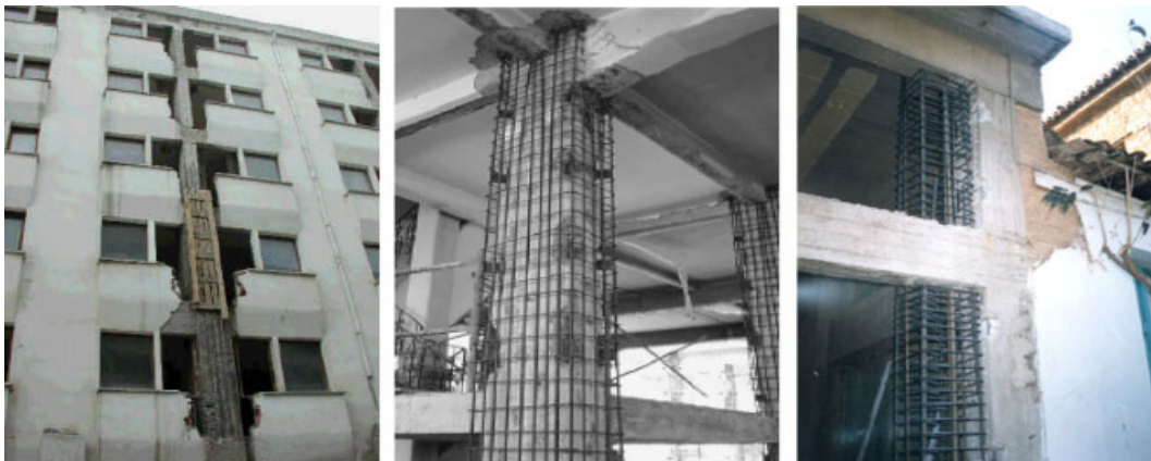
Fig. 4 Reinforced concrete jacketing technique
