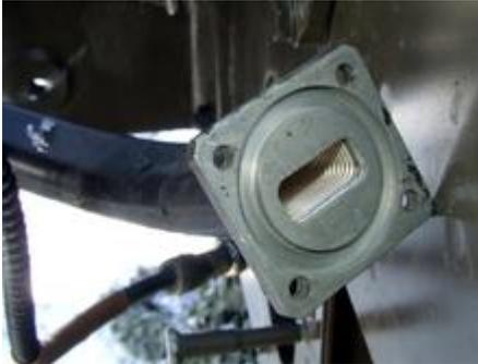
A section of flexible waveguide with apressurizable flange
