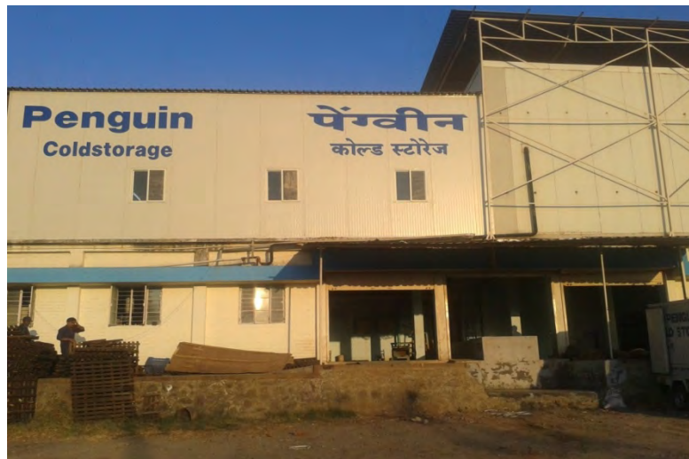
Figure 3 Penguin cold storage plant
