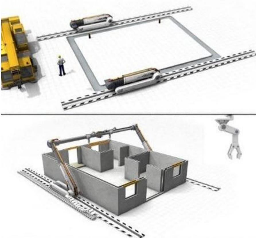
Contour crafting (CC) is a method of layered object manufacturing (LOM) process that uses polymer, ceramic slurry, cement, and a variety of other materials and mixes to build large scale objects with smooth surface finish.
