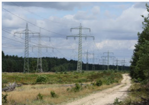
High-voltage transmission lines (HV OH lines) - Germany, Lower Saxony, Unterlüß
