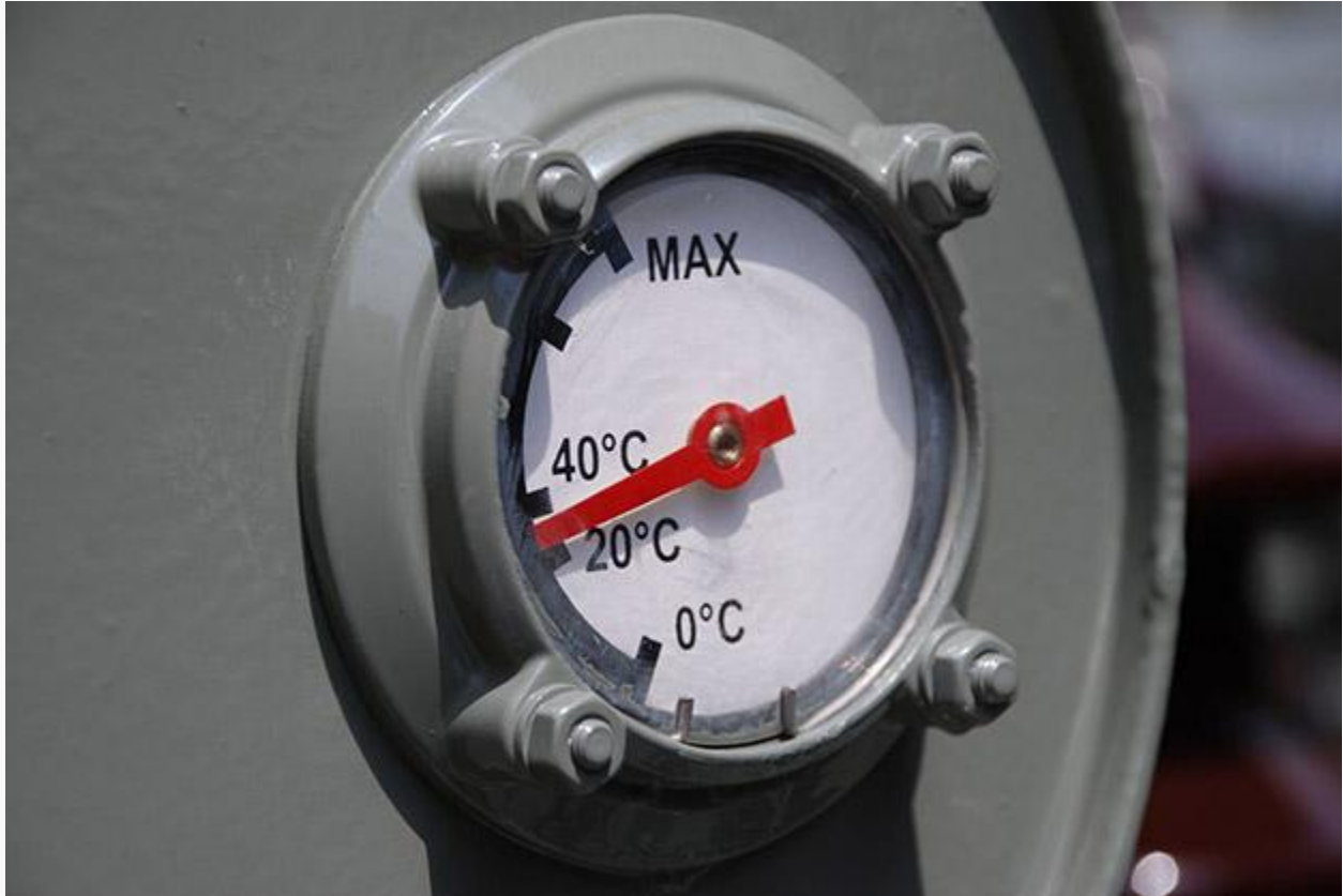
Transformer oil level indicator
