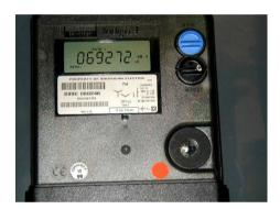
The reading for the meter shown is 069272.
