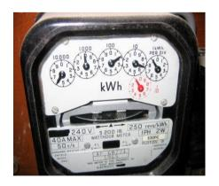
The reading for the meter shown is 94694.
