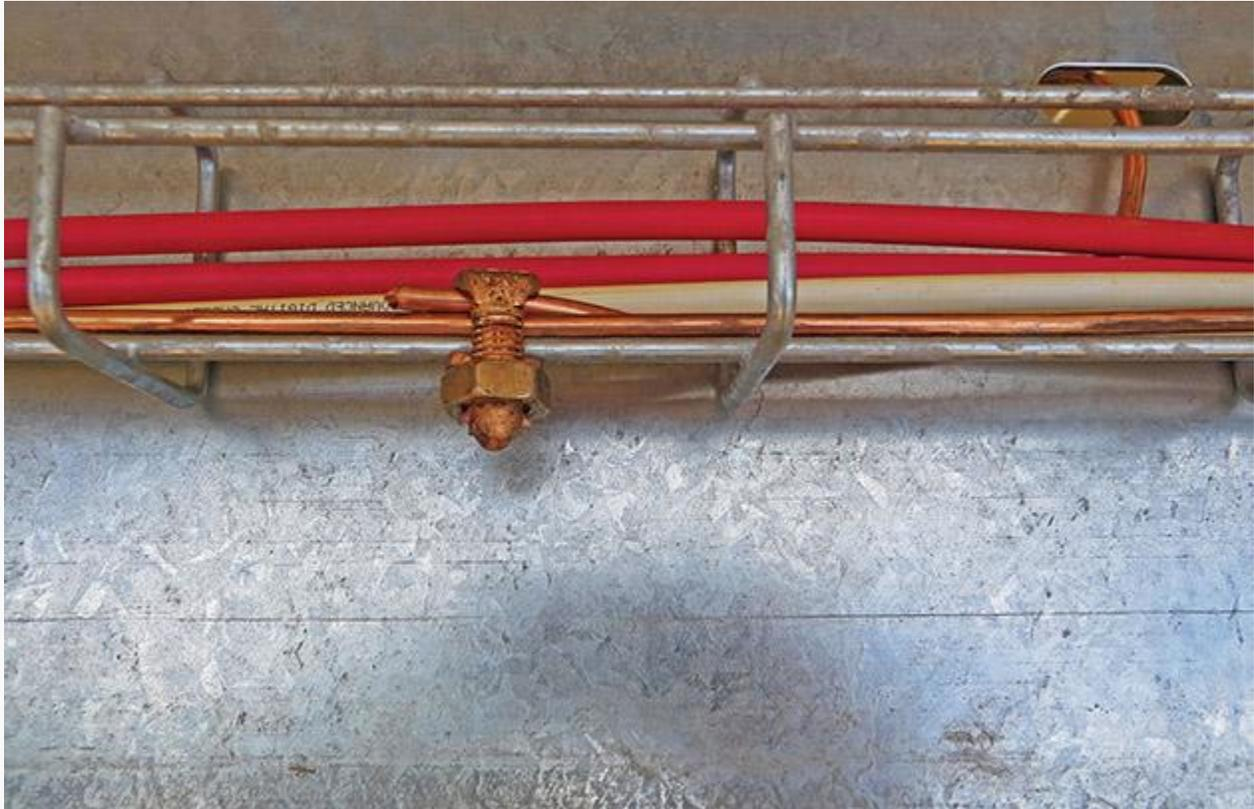
Grounding and bonding of cable trays (on photo: Ground wire connected to cable tray; photo credit: solarprofessional.com)
