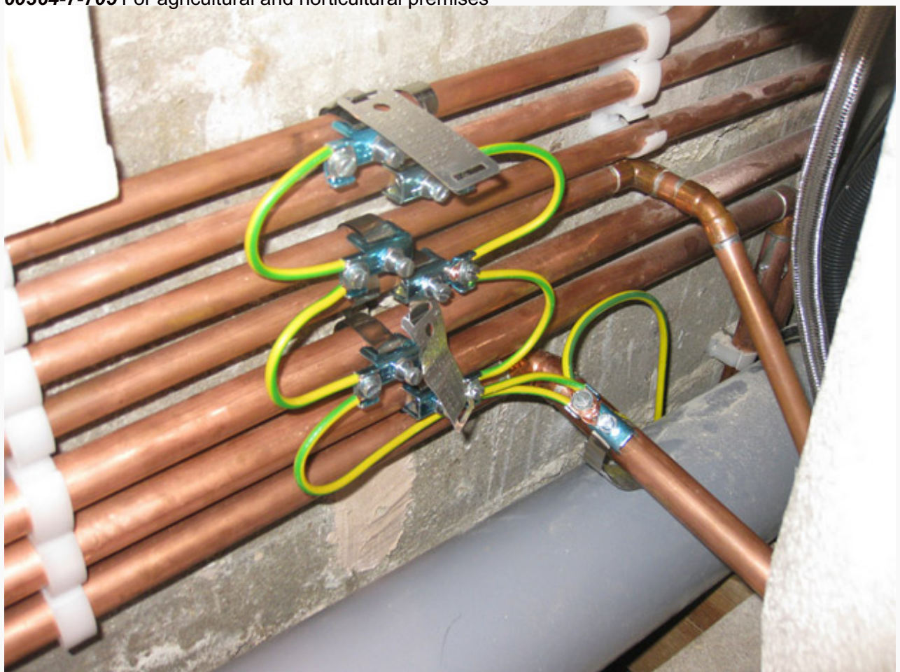
Figure 3 - Equipotential bonding of heating pipes
