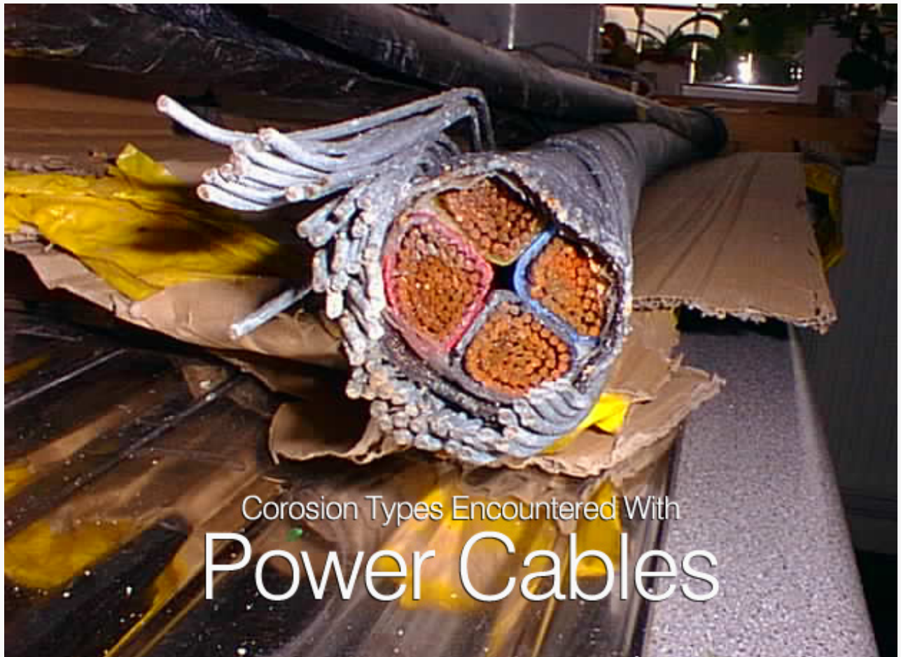
Corrosion Types Encountered With Power Cables
