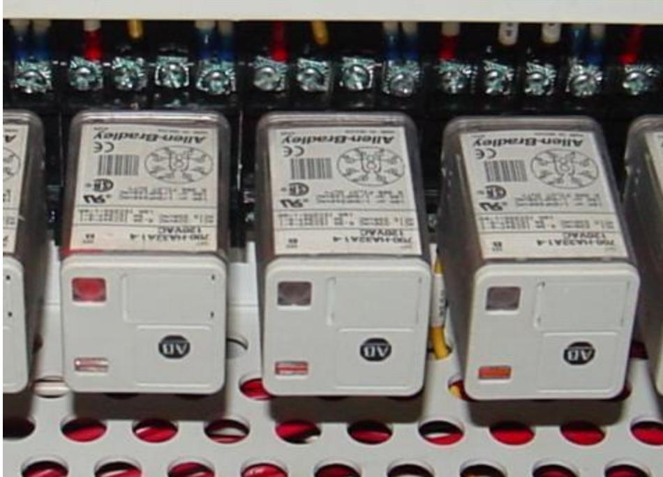
The relay units shown here are called "octal-base," because they plug into matching sockets, the electrical connections secured via eight metal pins on the relay bottom. The screw terminal connections you see in the photograph where wires connect to the relays are actually part of the socket assembly, into which each relay is plugged. This type of construction facilitates easy removal and replacement of the relay(s) in the event of failure.
