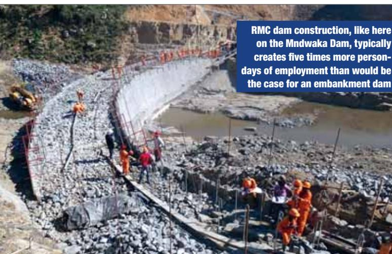
**RMC dam construction, like here on the Mndwaka Dam, typically creates five times more person-days of employment than would be the case for an embankment dam**
