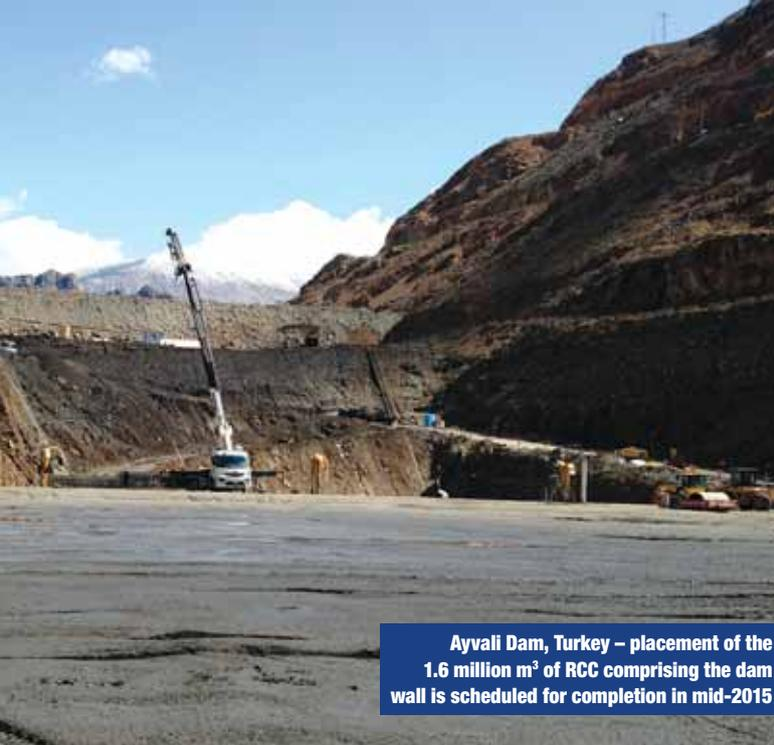
**Ayvali Dam, Turkey – placement of the 1.6 million m<sup>3</sup> of RCC comprising the dam wall is scheduled for completion in mid-2015**
