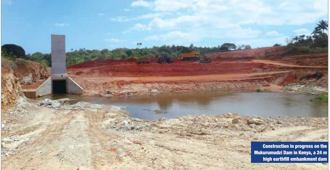
Construction in progress on the Mukurumudzi Dam in Kenya, a 24 m high earthfill embankment dam
