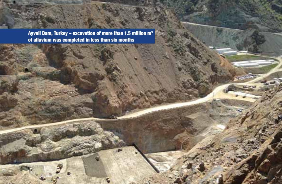
**Ayvali Dam, Turkey – excavation of more than 1.5 million m<sup>3</sup> of alluvium was completed in less than six months**
