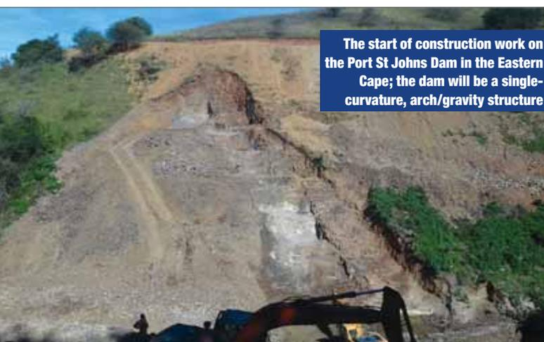
**The start of construction work on the Port St Johns Dam in the Eastern Cape; the dam will be a single-curvature, arch/gravity structure**
