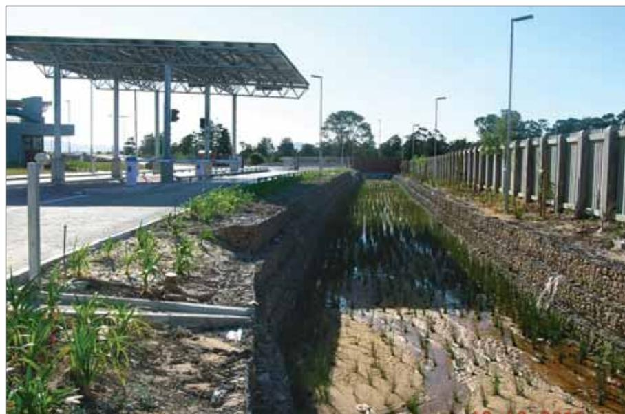
Figure 6 Trapezoidal cross-section of bio-swale with gabion side walls (October 2010); note vegetation sprigs
