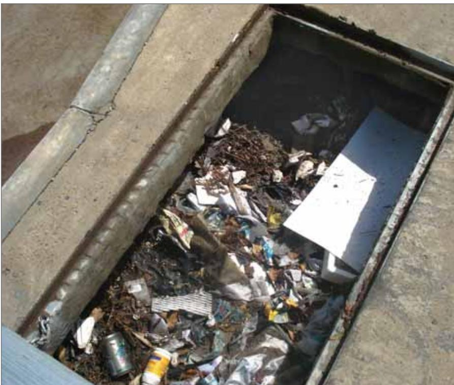
Figure 4 Settled litter, debris, silt and other particulates to be cleaned out (April 2012)
