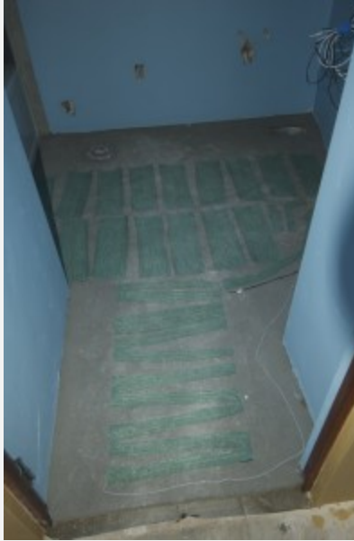
"Warmly Yours" electric heating mat being embedded in Natalie's bathroom floor
