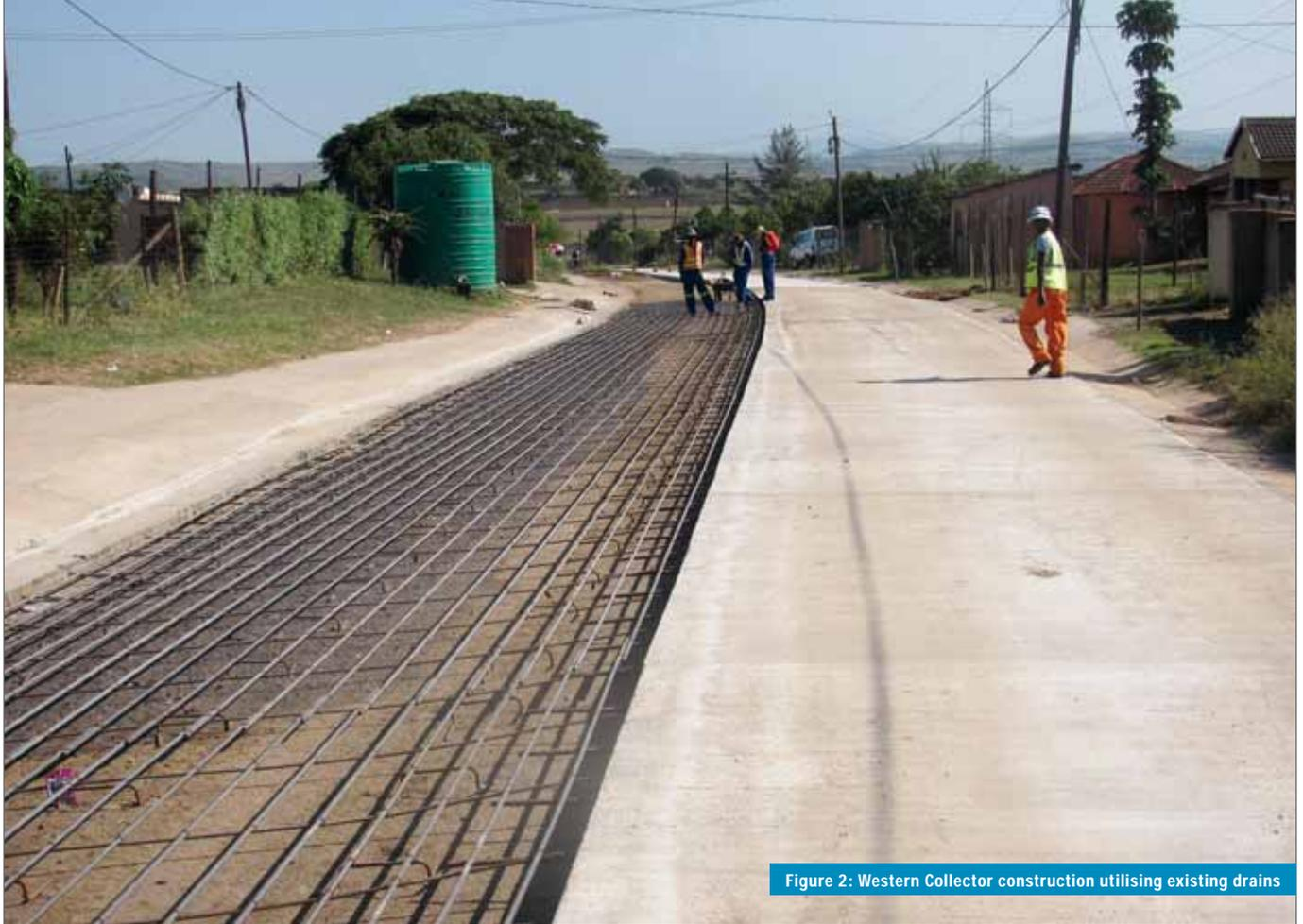
Figure 2: Western Collector construction utilising existing drains
