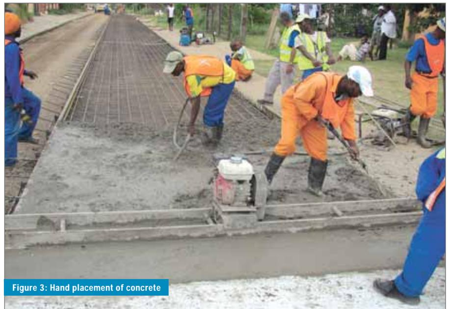
Figure 3: Hand placement of concrete
