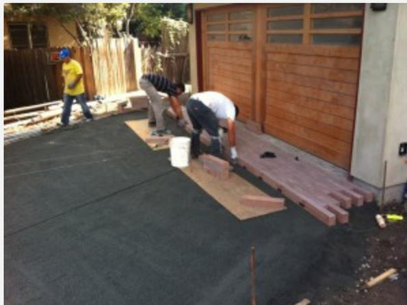
The driveway pavers being laid. We used 4"x18" pavers - the same aspect ratio used at Stanford at the CCSR building, and had them laid on the same orientation as the house so that they and the paving stones would all change your orientation to our "off kilter" house as soon as you stepped onto the property
