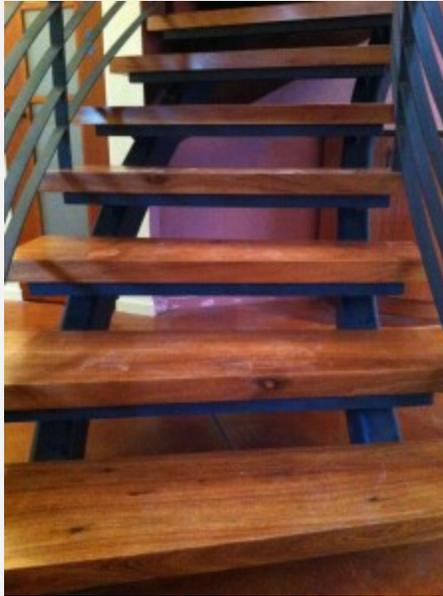
Black wooden strips secured to the underside of the stairs to narrow the space to that ever-so-critical-for-inspection smaller-than-baby-head size (and fortunately, the addition actually makes the steps seem to "float" even more than they did when you could see the supports)
