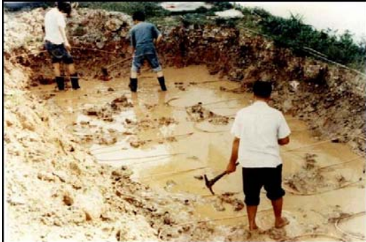
Fig. 2 Photograph of copper coil of the M-AC buried in the ground
