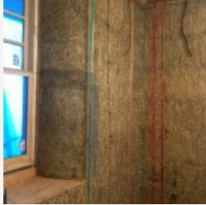
When finished, straw is tightly packed under the lath
