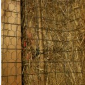
Close-up of corner
