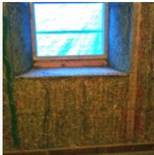
The window area -- ready for plaster
