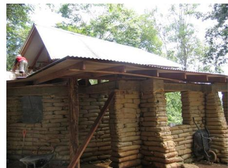
wall below. Overall it is a labor intensive process using hand tools. This simple and visually obvious process works well for one-story buildings, and can easily support upper levels.
