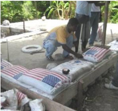
Geo-textiles are a high-tech way to make retaining structures, dams, and even airfields. Surprisingly, they also allow a very low-tech approach to buildings. Earthbag is a form of geo-textile building construction that is growing in popularity around the world. Recent engineering tests of the strength of different forms of earthbag
