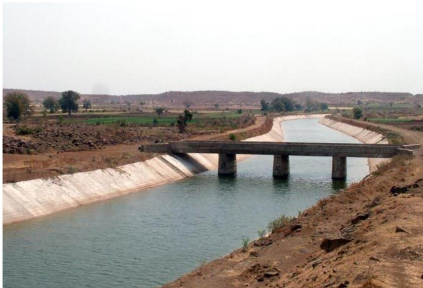
*The Narmada Main Canal is the largest irrigation lined canal in the world, supplying water at a capacity of 1,133 cubic metres a second. Image courtesy of Nvvchar.*
