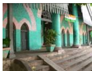
Fig. 10. View of the arches
