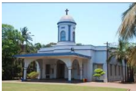
Fig. 5 Front view of St. John's Church
