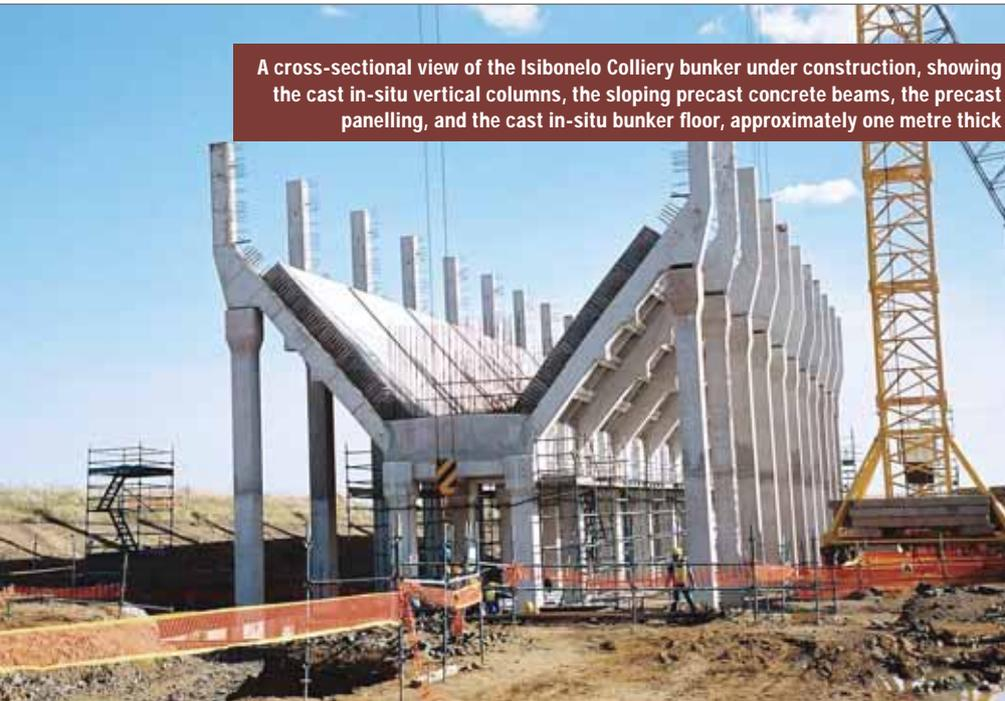
An external view of the Isibonelo Colliery bunker while still under construction, showing the vertical cast in-situ columns, precast concrete sloping beams and the precast panelling
