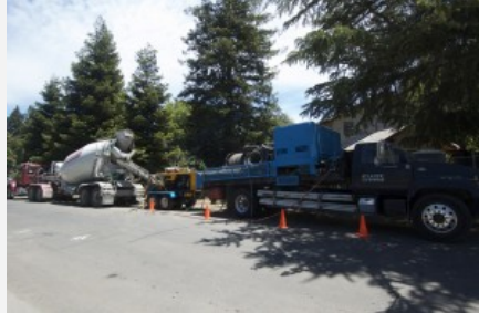
The guys from Atlantic concrete with the truck and the pump
