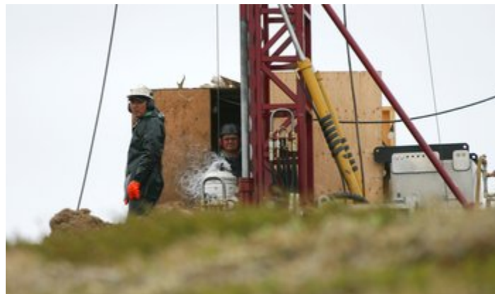
Workers and spurts of water at a drill rig, Pebble East.
