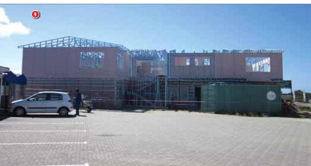
7 Steyns-Holzfaller shop and flats: composite slab made up of concrete and light-gauge steel joists
