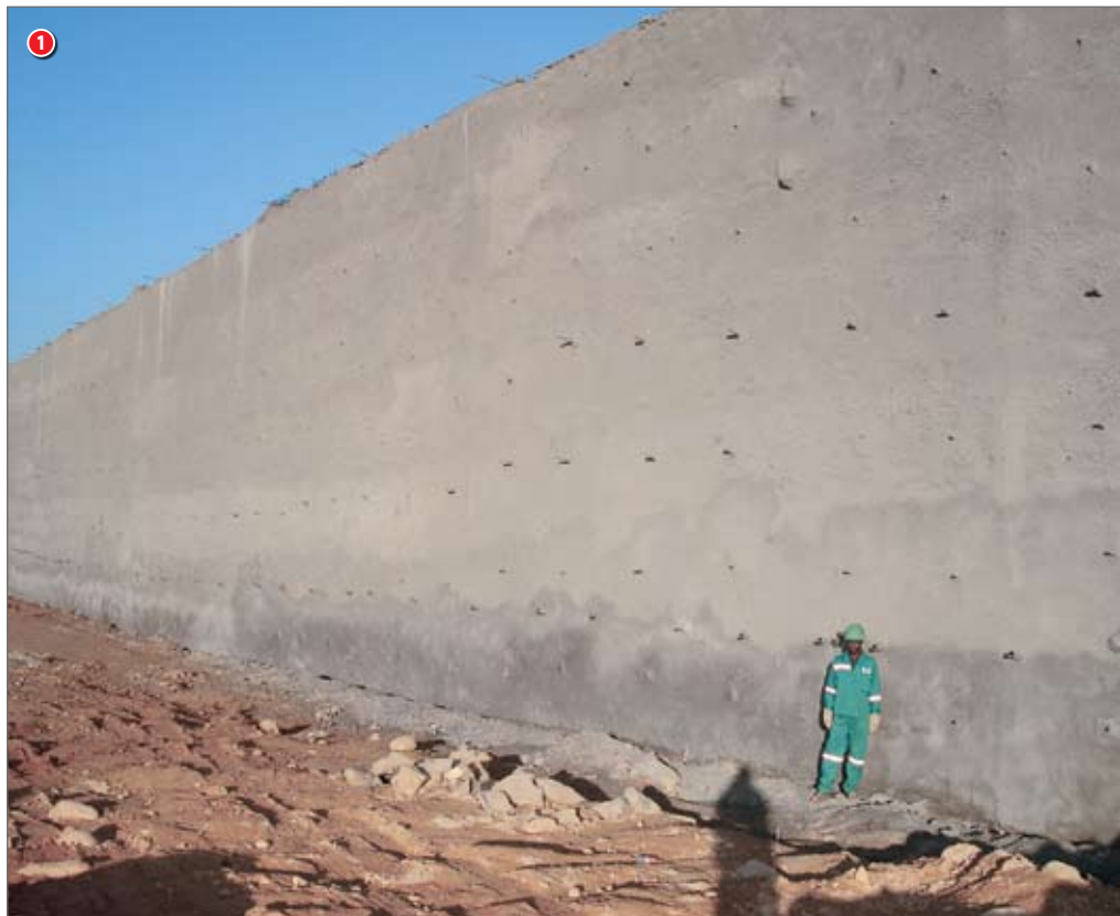
1 The site during the excavation phase
