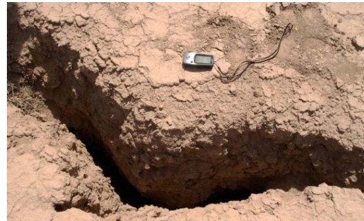
Fig. 5. Deep cracks in YA basin Eslamizadeh, A. 2009 [4]
