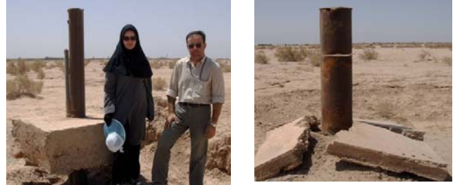
Fig. 4. The growth of water wells casing due to land subsidence
