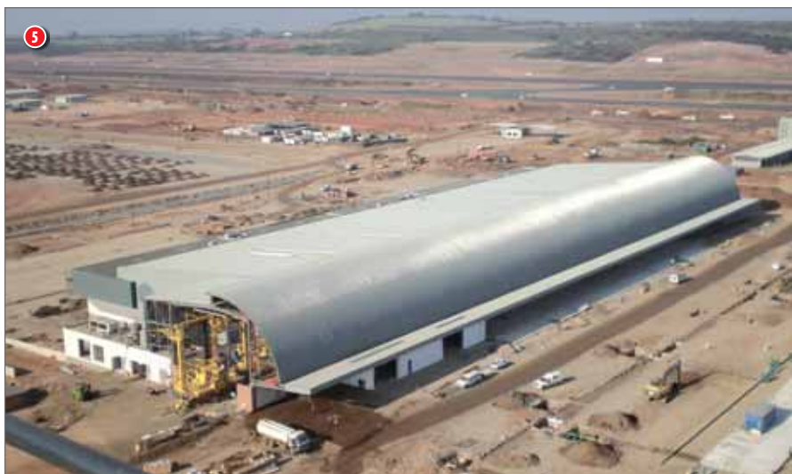
5 Completed cargo handling hall
