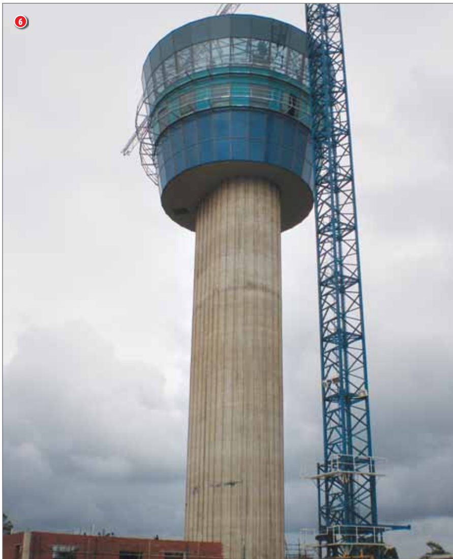
6 Control tower cab being erected
