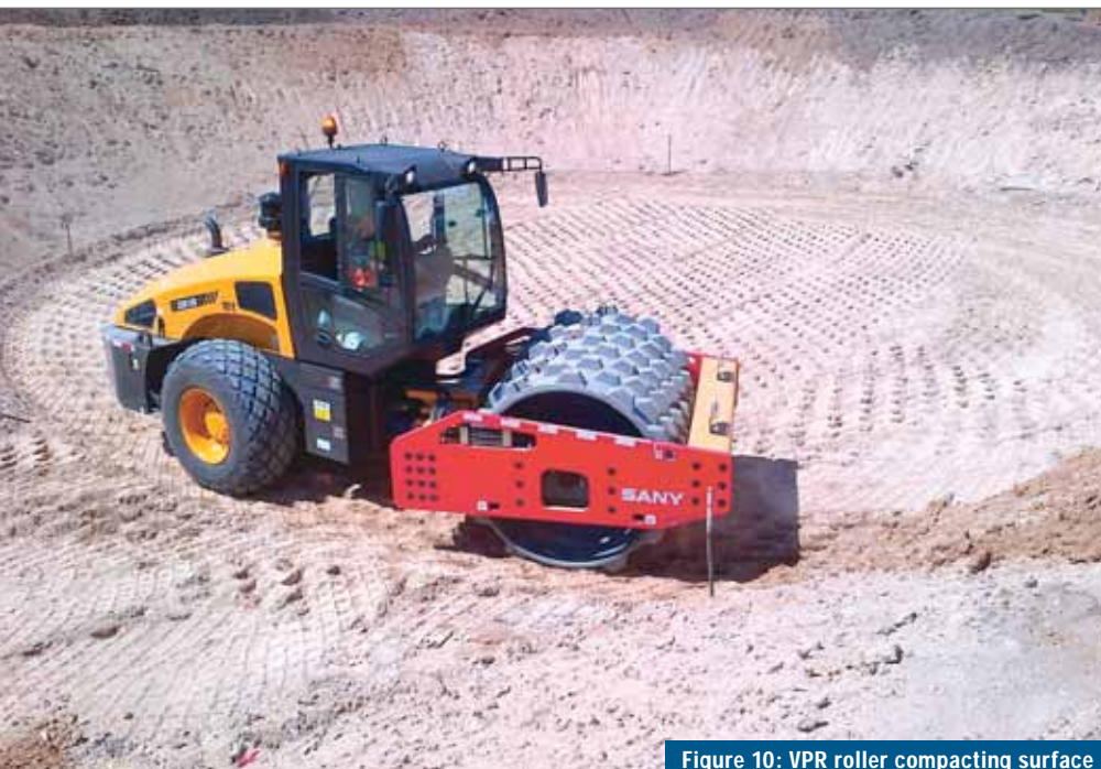
Figure 10: VPR roller compacting surface
