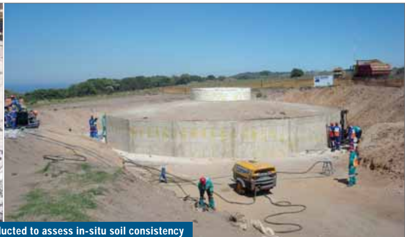
Figures 8 and 9: DPSH tests were conducted to assess in-situ soil consistency
