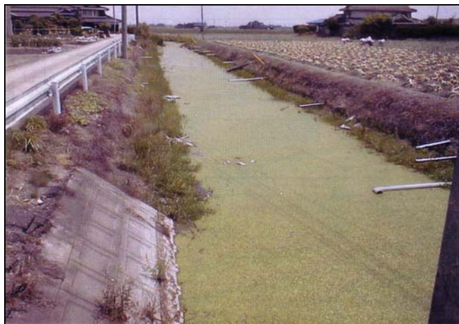
Fig. 13 Occurrence of Algae along the Interceptor Drains as a Results of Eutrophication
