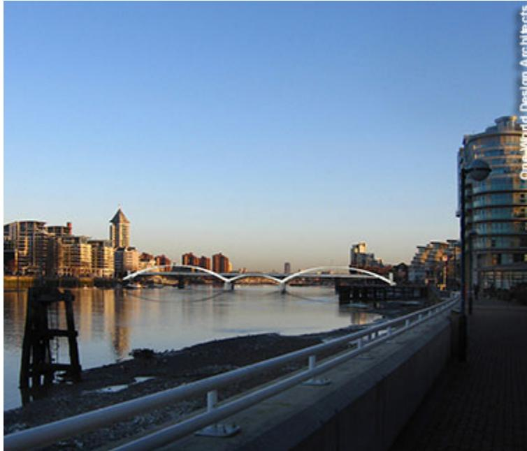
*A three-span footbridge planned to cross the River Thames has successfully passed through a second round of planning permissions. Two larger outer arches, which arc above the deck, are joined in the middle by a shorter, smaller arch that passes below the deck. One-World Design Architects*
