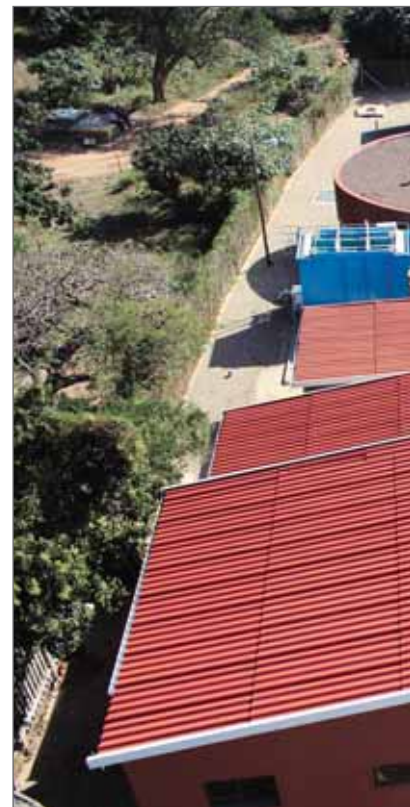
Photo 2: Raw water suction and high-lift delivery pump station at Shengeza Lake built into bank of lake with indigenous ground cover to follow
