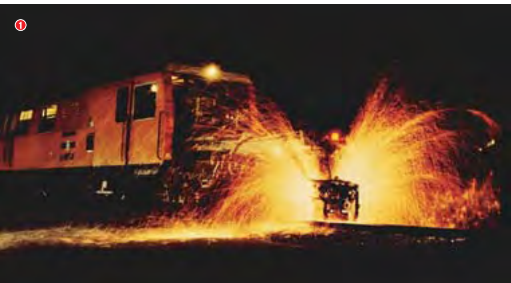
► Figure 1 Plasser & Theurer K355 APT flash butt welding machine Figure 2 Welding phases on printout Figure 3 Welding upset visible shortly after shearing
