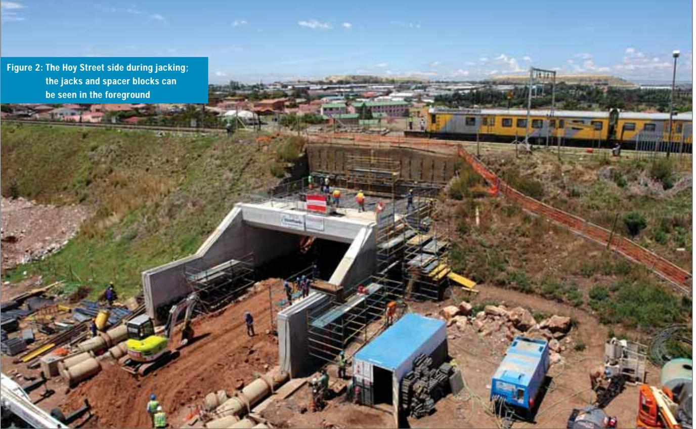
The drum-deck was constructed next. This activity used high-load capacity frames supplied by Doka. The top surface was power-floated in order to make the top surface as smooth as possible, and bentonite and HDPE sheets were used to keep the jacking friction coefficient as low as possible.
