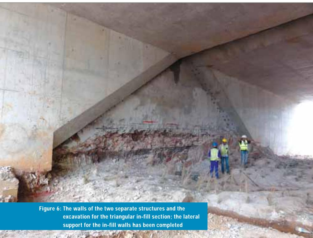
Figure 6: The walls of the two separate structures and the excavation for the triangular in-fill section; the lateral support for the in-fill walls has been completed
