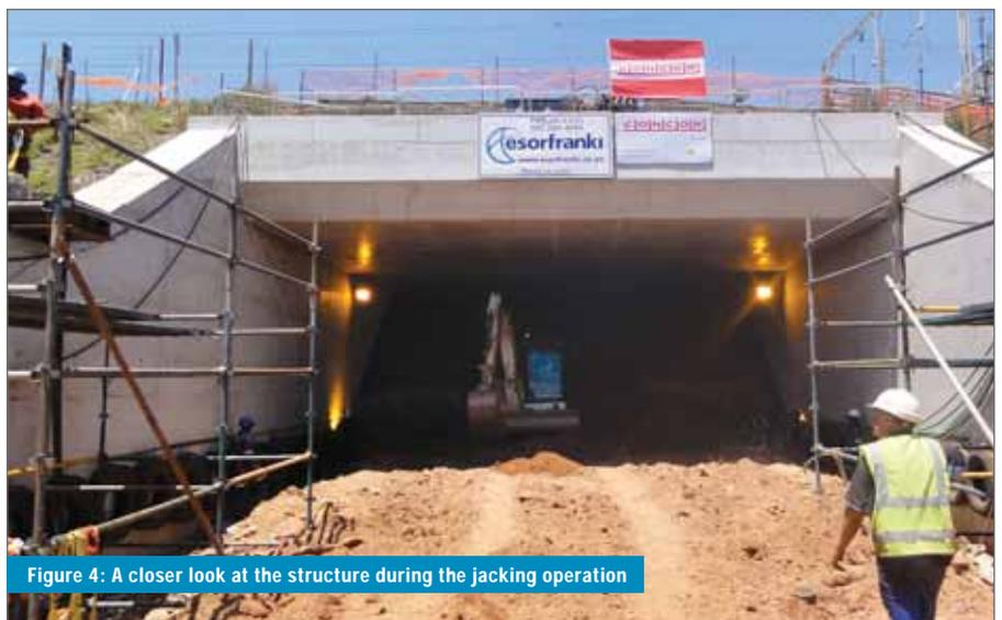
Figure 4: A closer look at the structure during the jacking operation
