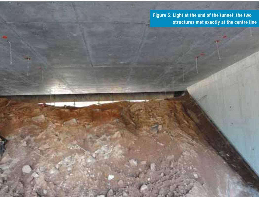
Figure 5: Light at the end of the tunnel; the two structures met exactly at the centre line
