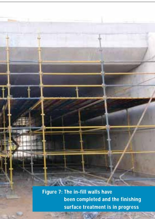
Figure 7: The in-fill walls have been completed and the finishing surface treatment is in progress
