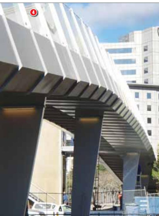
The compressive buckling resistance of the web plates was another important design consideration. Using a plate model, the stresses in the webs were calculated and verified using hand calculations. In this instance the 10 mm transverse diaphragms, provided at approximately 2 m centres, help restrain the web panels against local buckling. These diaphragms also prevent the distortion of the box girder under the applied torsional stresses.
