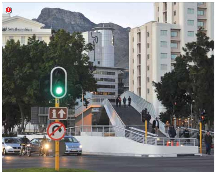
The bridge is unconventional in that it incorporates items such as lift shafts, architectural lighting, glazing and CCTV. The successful integration of these items into the design and during construction required careful coordination on a technical and architectural level. A review and approval process was therefore put in place so that each member of the professional team could be informed about the design development of the various components on the bridge.
