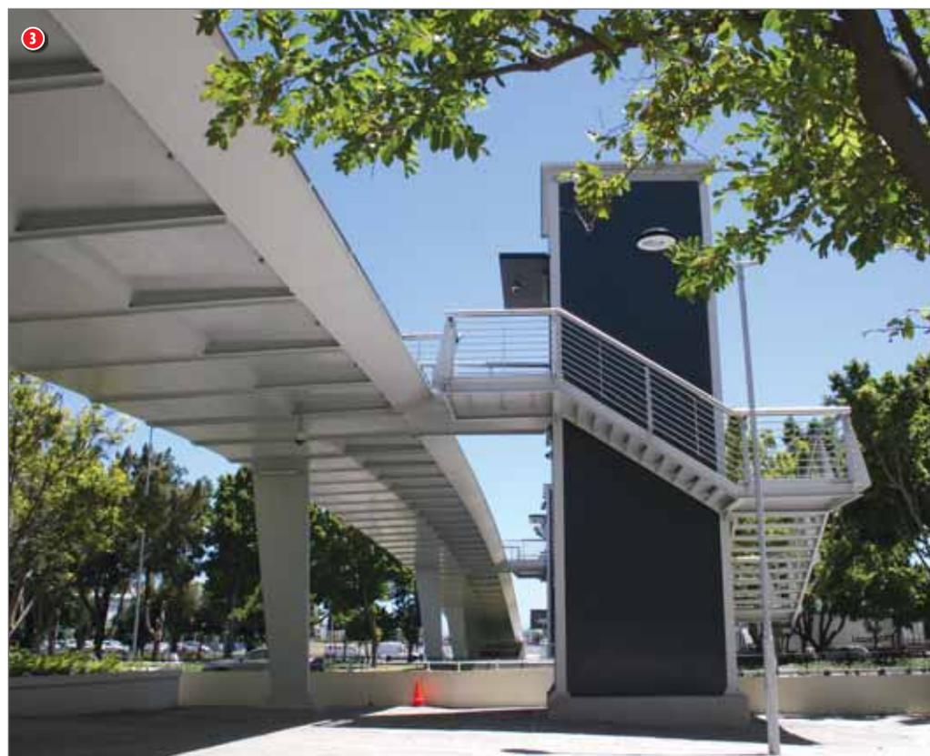
it to taper geometrically towards its base. The end result is unique and aesthetically pleasing, and in harmony with the asymmetric deck section.
