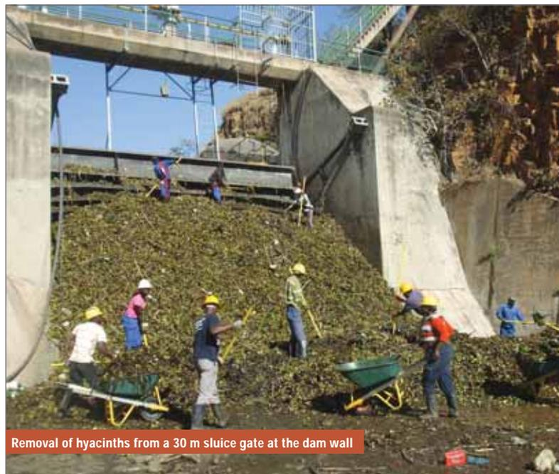
impact on the greater environment, often affecting bird- and other wildlife, as well as posing a danger to recreational users of the dam. Debris containment curtains are constructed at the Crocodile River inlet to the dam, and during periods of normal rainfall most of the debris is trapped and successfully removed.
