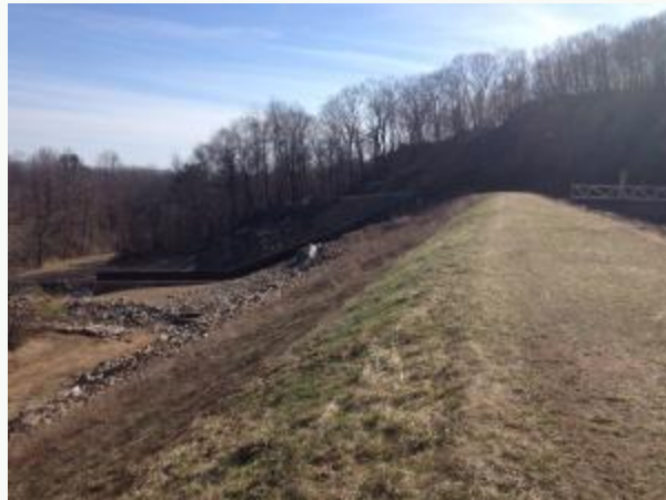
The dam with spillway on the other end.
