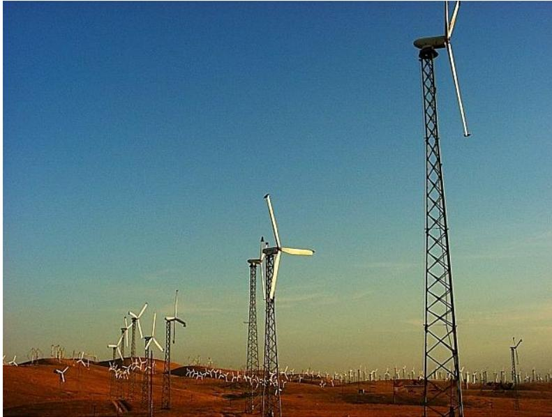
Older style wind turbine towers using latticing at Altamont Pass, California.
