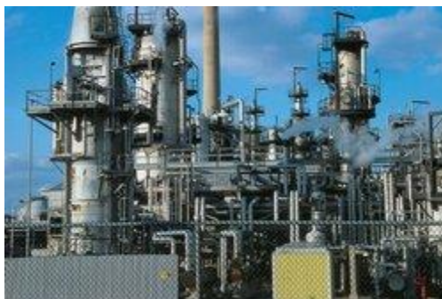
Oil refinery. Photo: DOE
