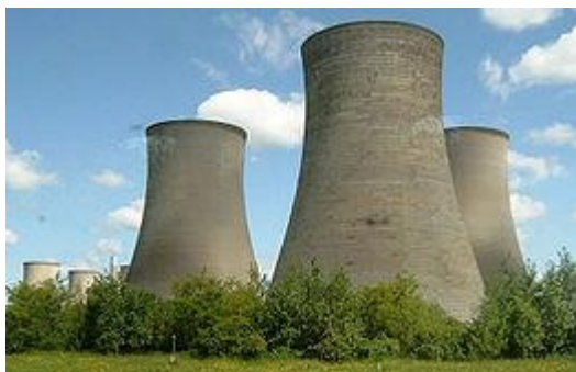
Hyperbolic cooling towers, Didcot fossil fuel power station, Oxfordshire, England.
