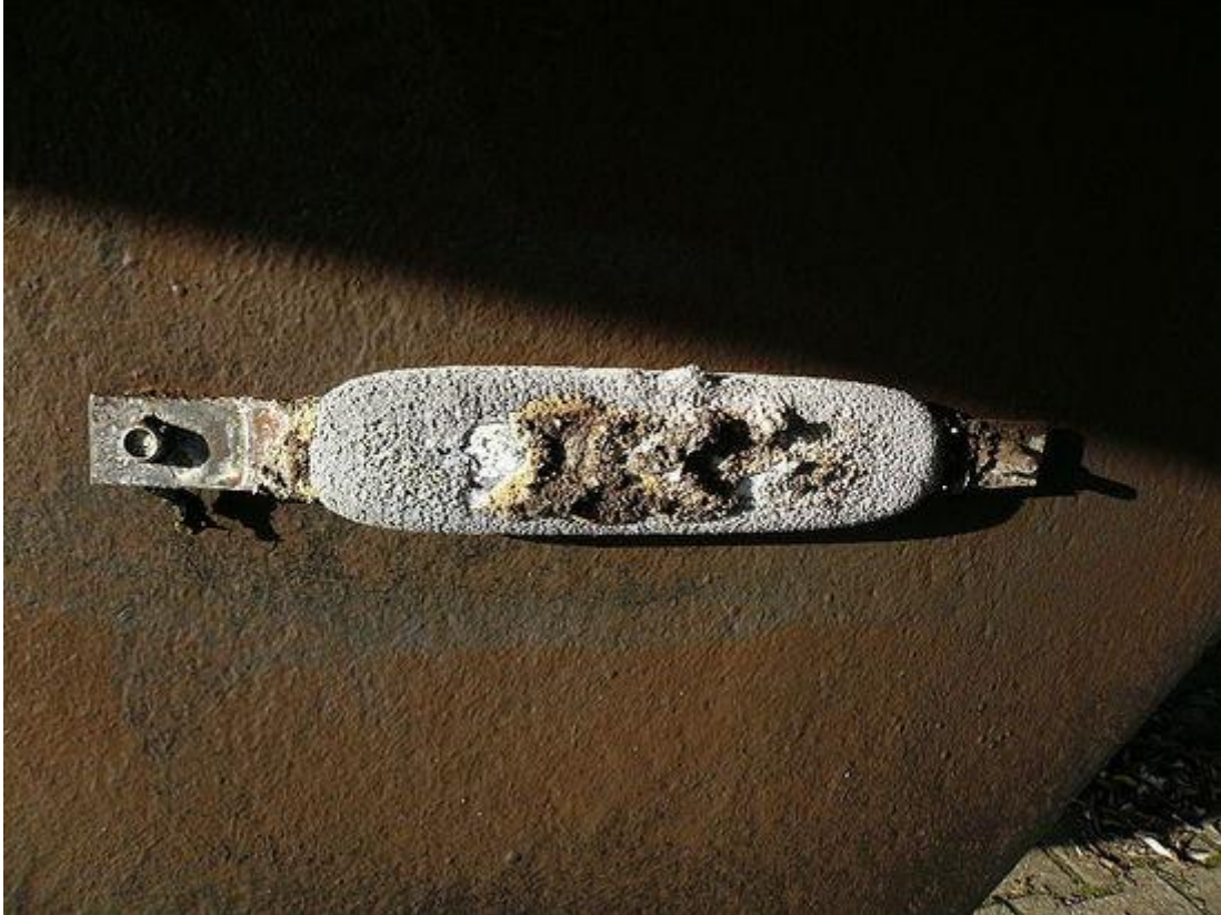
Figure 1. Partially corroded sacrificial anode on the hull of a ship. Figures courtesy of Wikipedia
