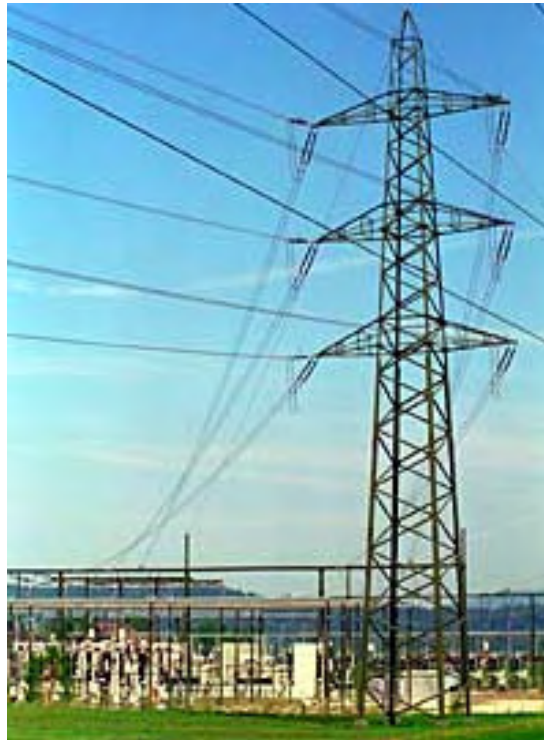
Figure 1.1 Typical view of an overhead transmission line terminating at a substation
