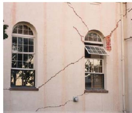
Figure 1. Crack pattern of masonry wall subjected to seismic event.
