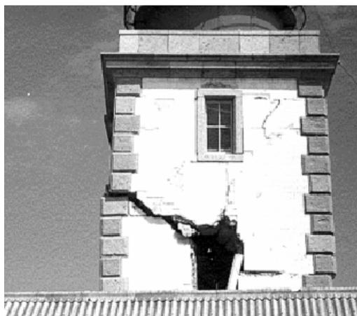
Figure 2. Crack pattern of masonry bell tower subjected to seismic event.
