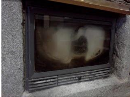
Image: Cassette flush with heat fans with 85% yield
