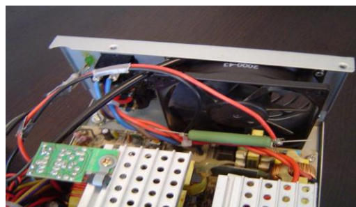
Minimum load installed close to fan.
