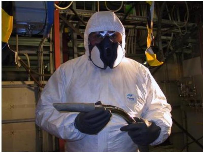
**Fig. 9:** Staff wearing protective clothing during work at  $SF_6$  waveguides
