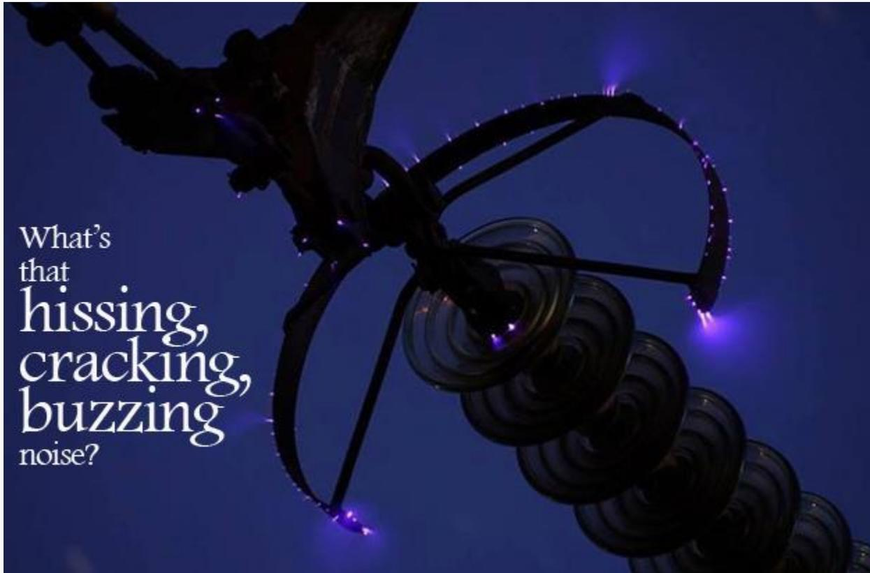
What's that hissing, cracking, buzzing noise? (on photo: Corona discharge on insulator string of a 500 kV transmission line)
