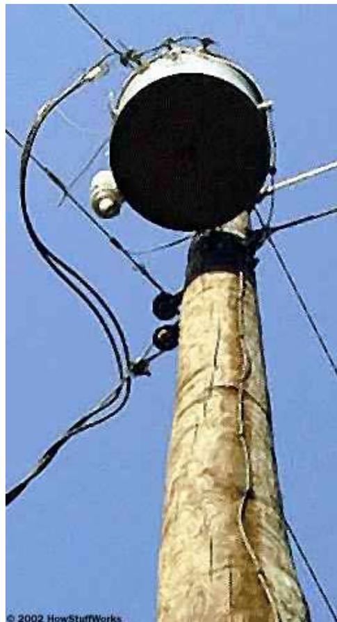
Every utility pole on the planet has a bare wire like this. If you ever watch the power company install a new pole, you will see that the end of that bare wire is stapled in a coil to the base of the pole. That coil
