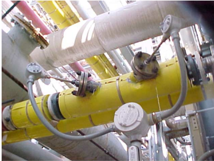
Fig. 6. Installation of Ultrasonic Transducers on 3" Titanium Pipe Measuring a Vent Stream with Continuously Varying Gas Composition to Throx Unit
