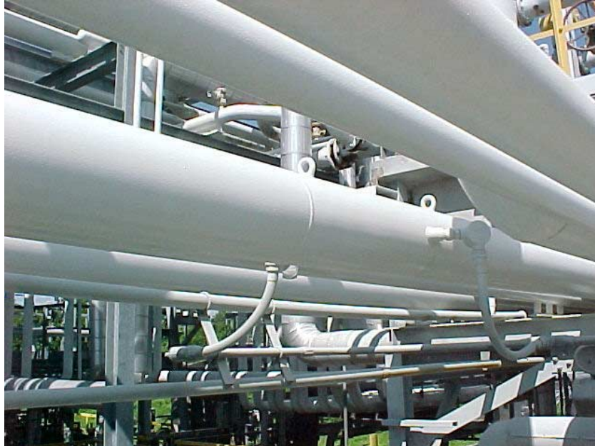
Fig. 3. Installation of Ultrasonic Transducers on 10" CS Pipe Transporting Flammable Liquid from Barge to Storage Tank
