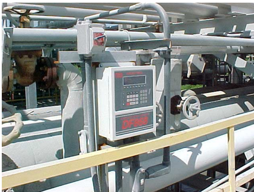
Fig. 2. Installation of DF868 Electronics
