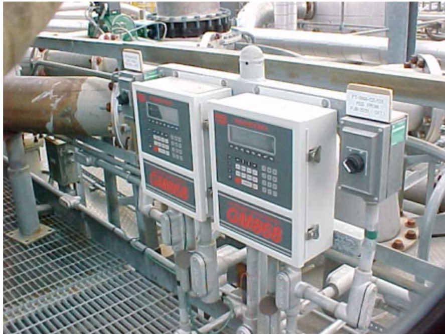
Fig. 4. Installation of Two Consoles, Each Containing GM868 Electronics
