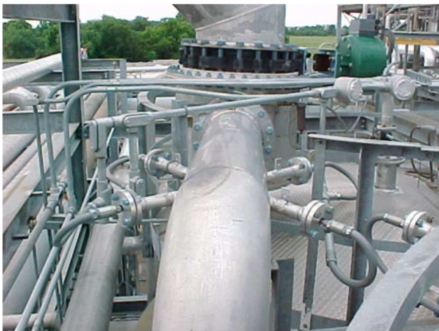
Fig. 5. Installation of Two-Path Ultrasonic Transducers on 16" Aluminum Pipe Measuring Bi-Directional Flow
