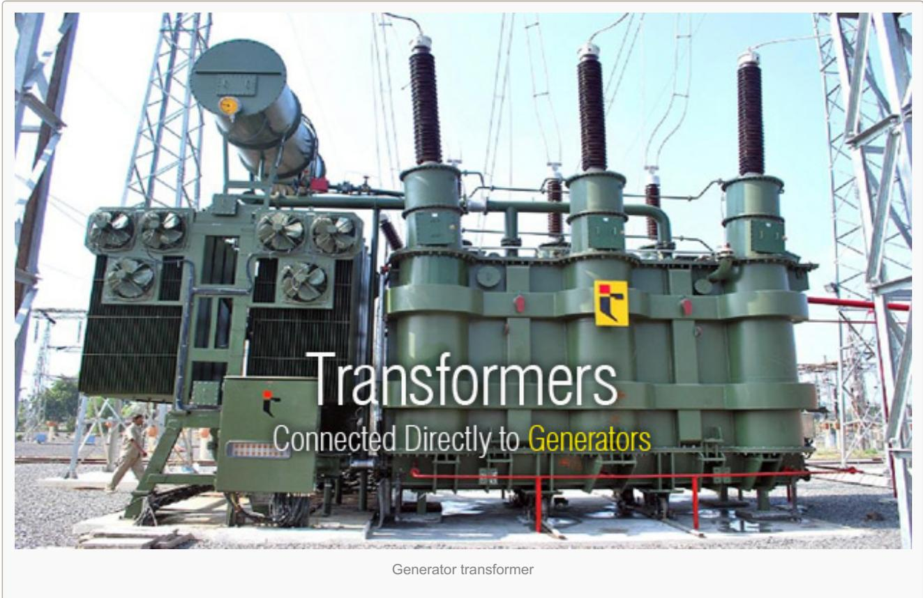
Power transformers connected directly to generators can experience excitation and short-circuit conditions beyond the requirements defined by [ANSI/IEEE standards](#). Special design considerations may be necessary to ensure that a power transformer is capable of withstanding the **abnormal thermal** and **mechanical aspects** that such conditions can create.
